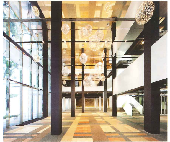
Contrasting infill glass building uses structural frame of earlier building
