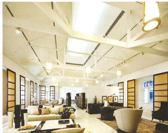
Exposed timber trusses in bungalow's soaring roof
