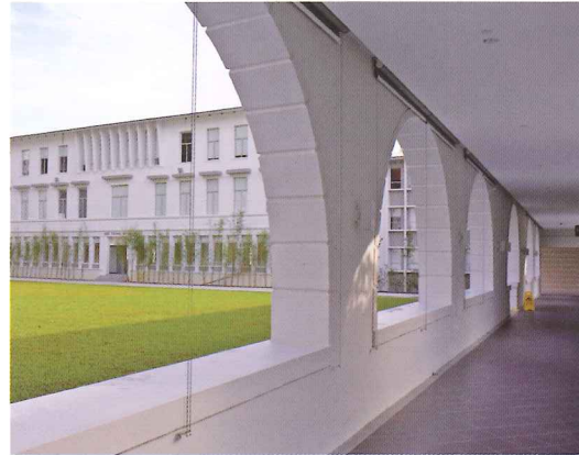
Cloistered passageway with rhythmic semi-circular openings
