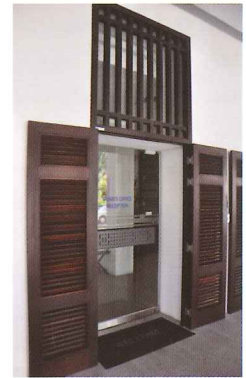
Timber lattice fanlight and louvered door
