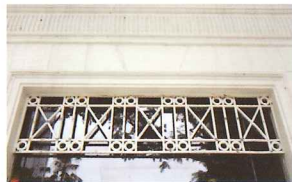
Fanlight grille at first storey
