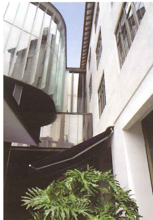
Recessed glass link between new and old
