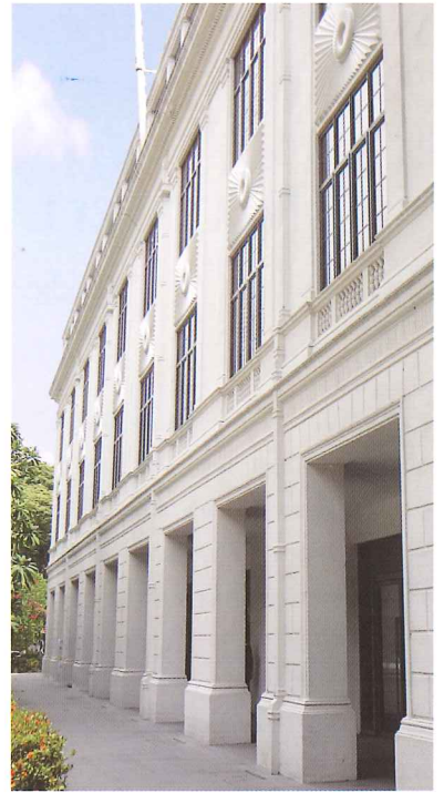
Former façade with rhythmic columns and rusticated finish
