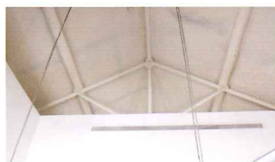
Original steel roof trusses
