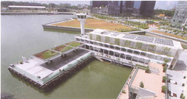
View of Customs House and pavilion
