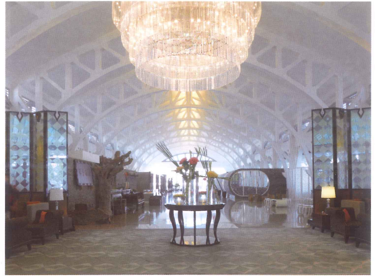
Clifford Pier's voluminous interior with concrete arched trusses
