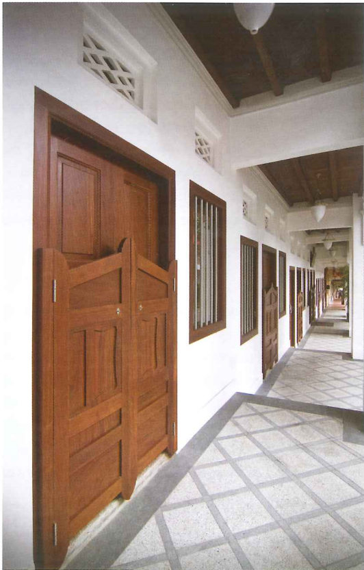
Pintu pagar of original design reinstated
