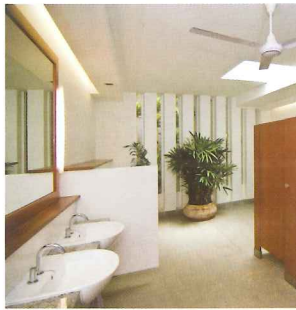
Vertical slot openings in restroom for natural lighting
