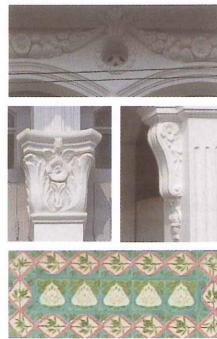
Key architectural elements restored
