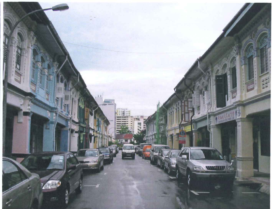
street view of conservation shophouses along lorong 24a geylang
