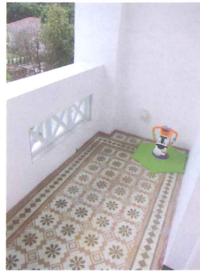
Original patterned floor tiles at second storey balcony
