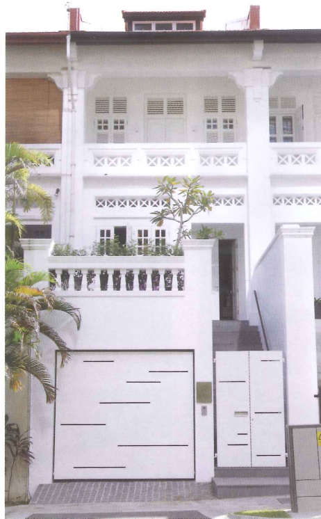
Restored terrace house with garage under the front terrace
