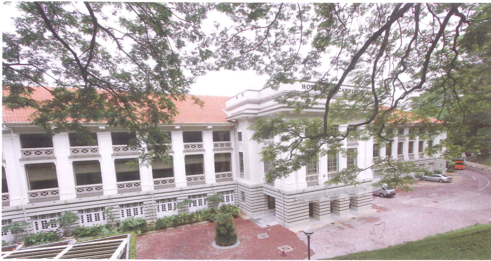
Original façade beautifully preserved
