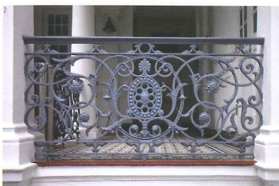
Cast iron railing
