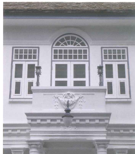
Close-up external architectural features
