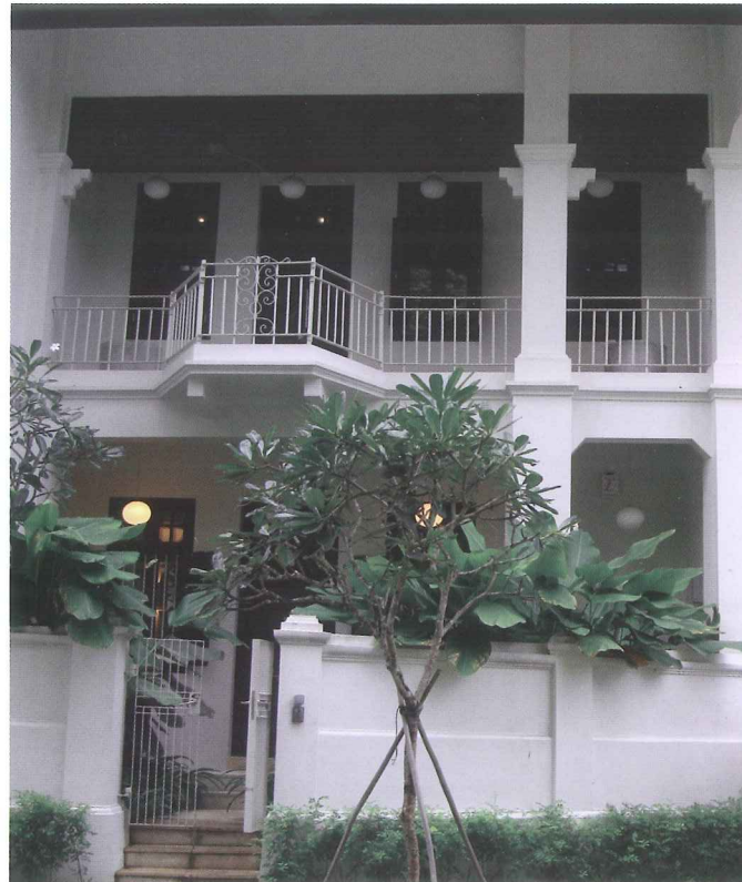
Art Deco terrace house restored into spacious family home
