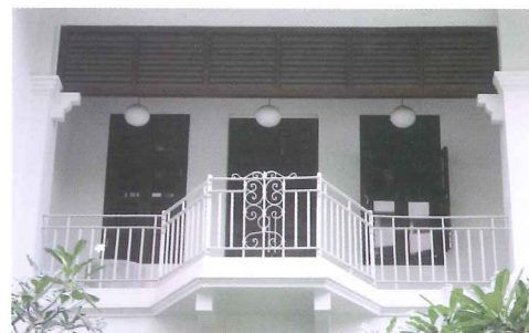
Cantilevered balcony with original railing design
