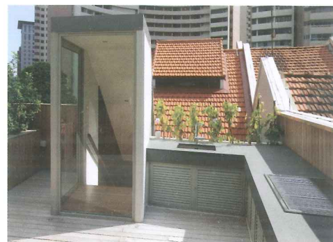
New staircase leading to roof terrace
