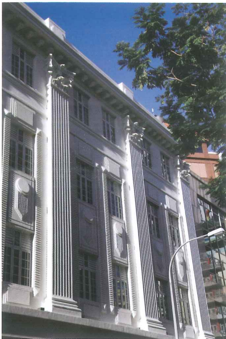
Restored façade of 36 Armenian Street
