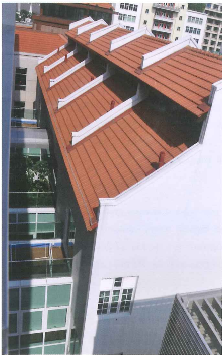
Original pitched roofs with firewall
