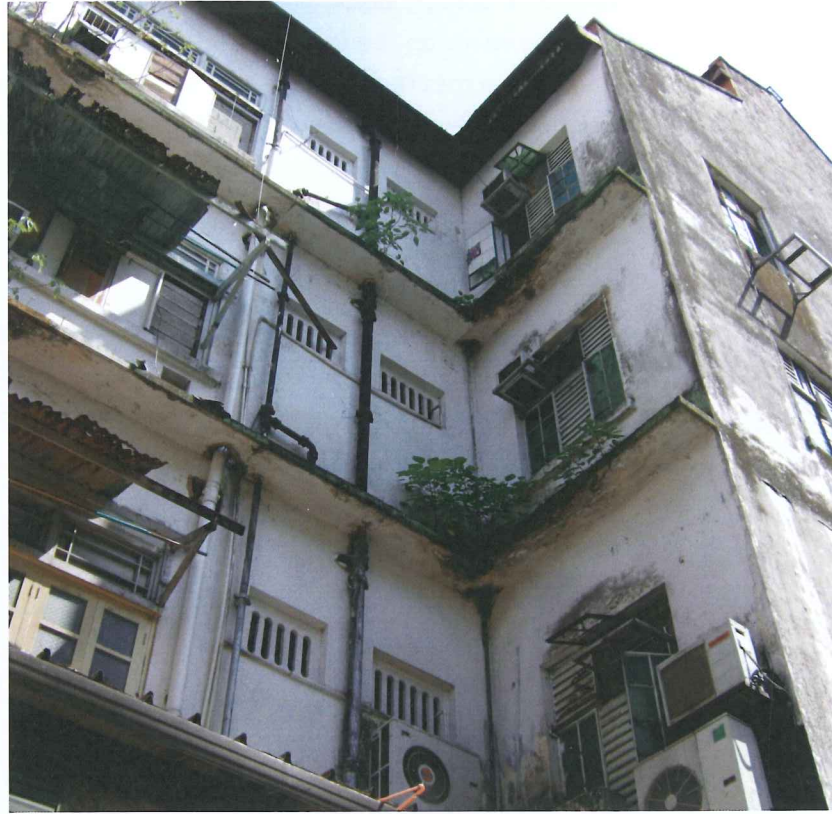
Figure 5: Existing rear of shophouse
