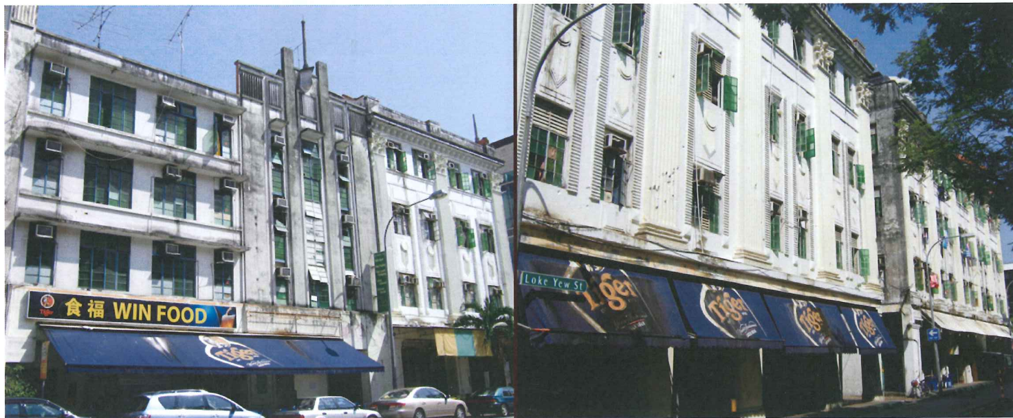
Figure 3: Condition of the existing conservation façade
