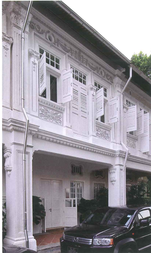
Terrace house restored with subtle charm
