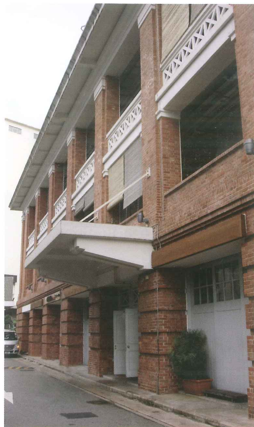
Side facade with concrete canopy
