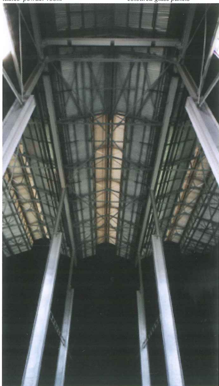
Exposed roof trusses and steel structures
