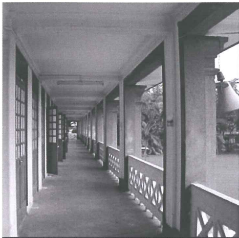
Corridor with well detailed cornices, columns, capitals & cross - Braced parapets
