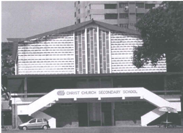
Front of hall-cum-canteen block with feature window and cantilevered dog-leg stairs
