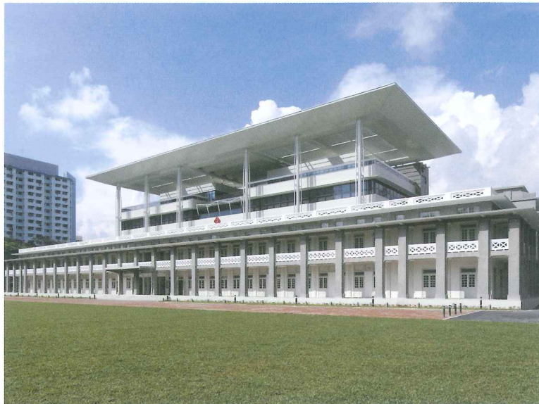
1933 school building restored with new five-storey extension at rear
