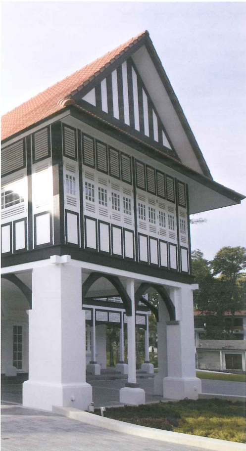
Decorative arch moulding & timber bracing at front porch
