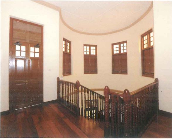
Timber door, windows and floor at second storey
