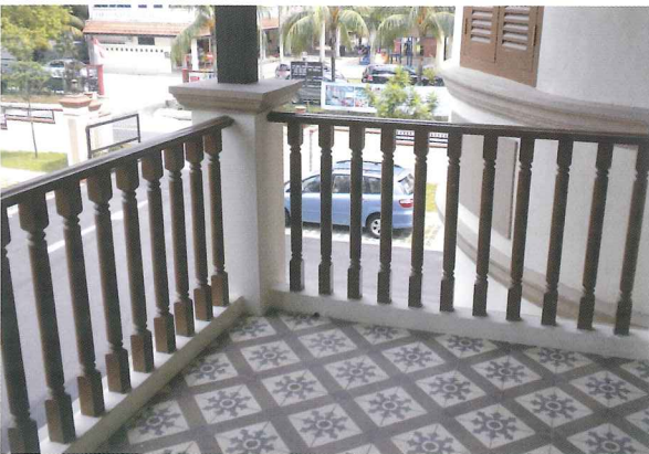
Timber balustrades retained
