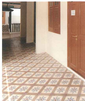
Original terrazzo floor tiles salvaged and reused
