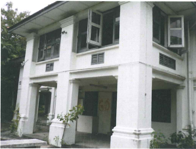
Fig 2.4 front view of entrance foyer
