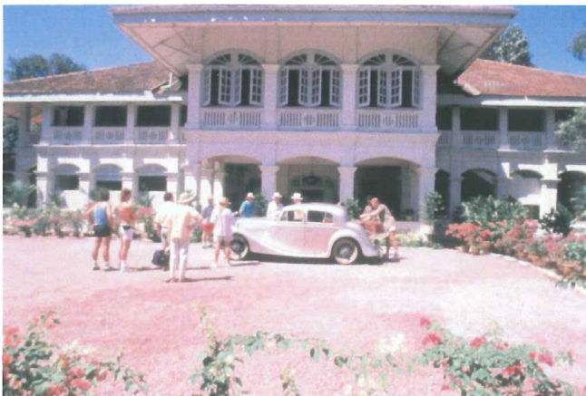
Fig 2.2 Block 48 with the additional windows and staircase added.
