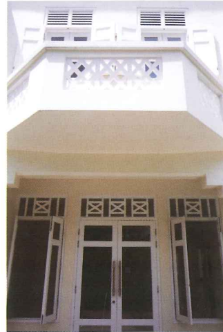
First storey façade with perforated parapet at protruding balcony above
