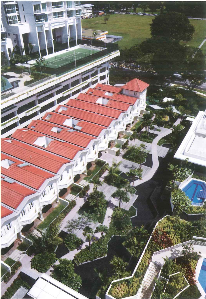
Aerial view of integrated old and new development with attractive landscape and water features
