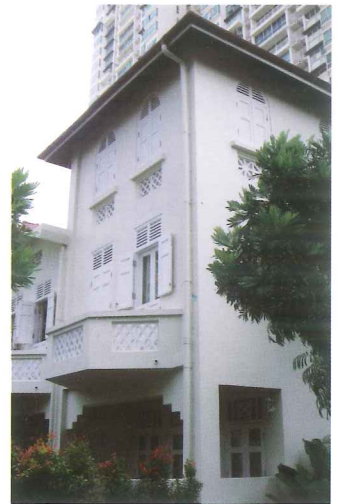
Façade of corner unit
