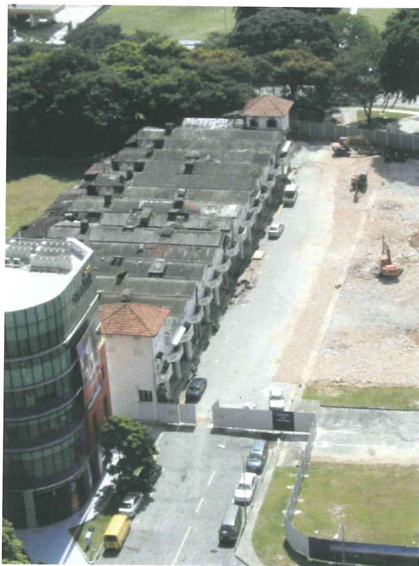
Jellicoe Road Shoohouses before conservation
