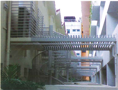
New circulatory and service elements integrated within rear courts
