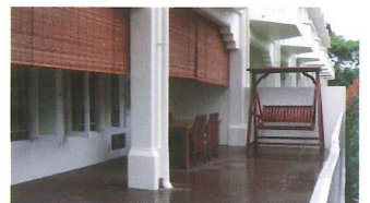
Previous walkway space converted to new terrace space
