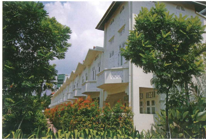
Double and triple storey shophouses restored into modern premium homes
