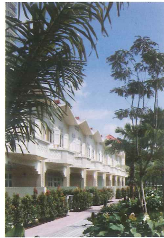
Zig-zag gabled roof and façade detailing repaired and restored
