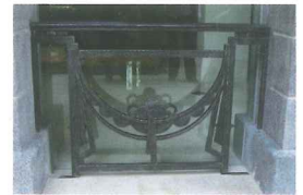
Restored cast-iron balustrade at first storey verandah
