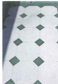
Original terrazzo floor finishes at second storey verandahs retained
