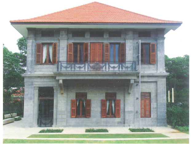
The restored bungalow
