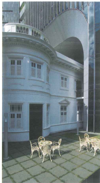
New residential tower cantilevered over restored bungalow
