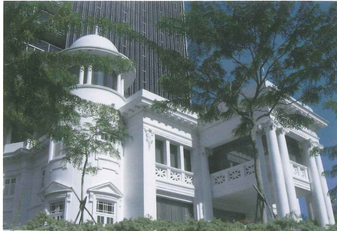
1930s bungalow with new 20-storey residential tower
