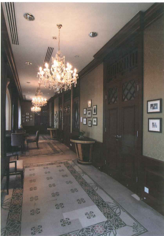
Peranakan cement tiles kept with damaged ones replaced
