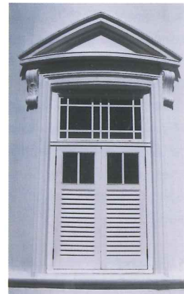
Original window with plaster triangular pediment above
