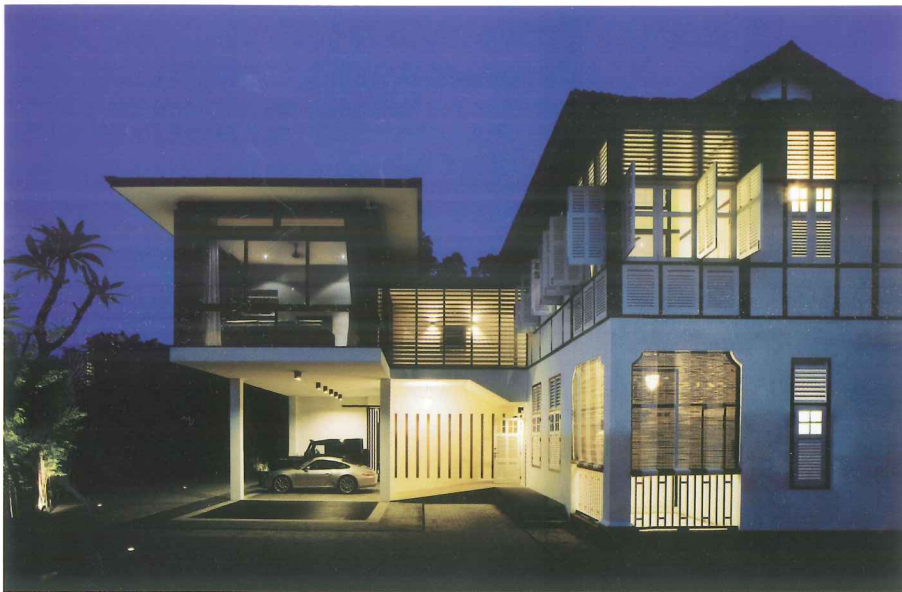
Linkway with adjustable louvred windows seamlessly connects the old and new buildings
