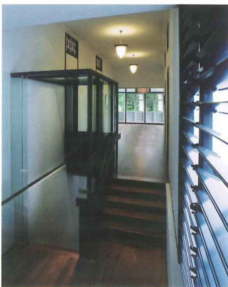
Glass box over staircase for better security to second storey
