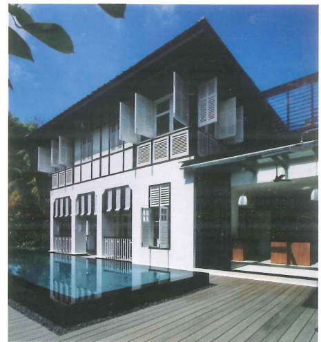
Conserved house seen from the raised pool deck in the foreground
