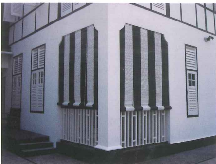
Existing railing kept
