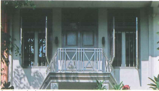
Second storey façade retained
