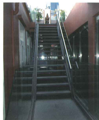
New access staircase at third storey to roof terrace and full height fire insulated glass panels to the right
