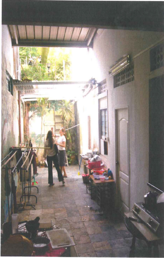
Image showing courtyard prior to restoration
