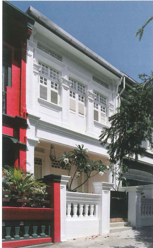
Maximum retention of terrace house as residence
