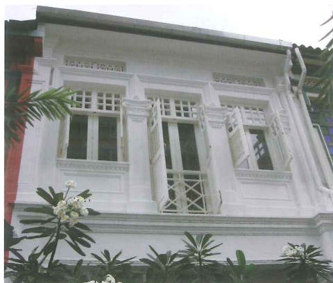
Timber windows retained and restored
