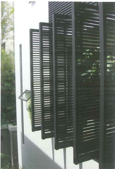
Timber louvred screens for privacy and natural lighting at second storey
