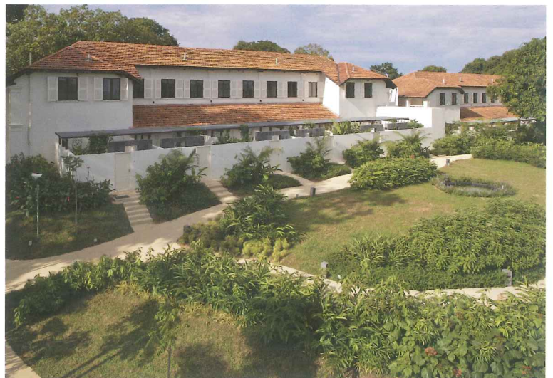
Landscaped garden at rear of restored army barracks
