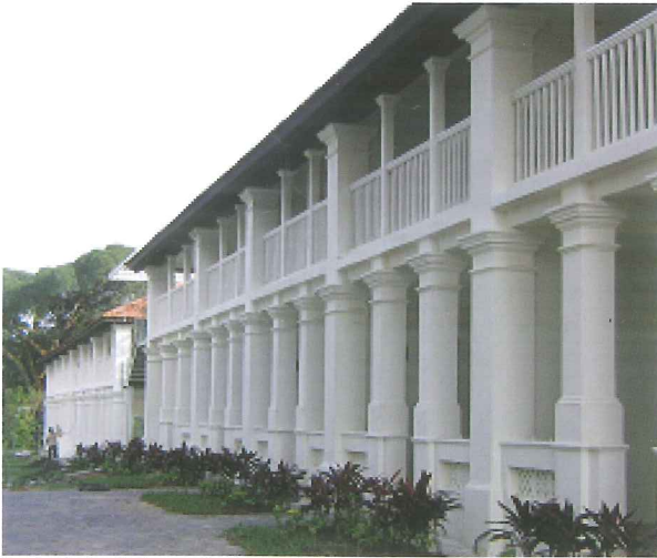
Regular rhythm of columns at first storey and original design of railing at second storey
