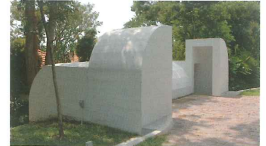
Existing air raid shelters retained
