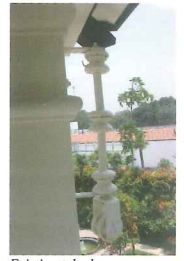
Existing telephone post kept
