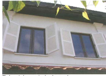
Timber windows retained and restored
