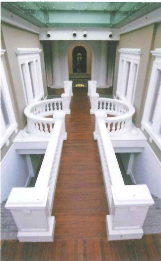
Seamless timber floor finish matching second storey central circulation
