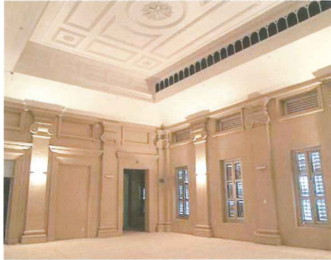
Decorative ceiling and pilasters kept
