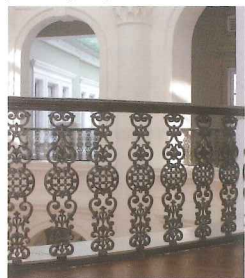
Balustrade at second storey stripped of paint and given coat of varnish
