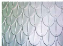
Unique zinc fish-scale tiles repaired and spray-painted
