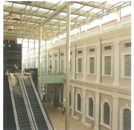
Contrast between modern and heavy masonry construction
