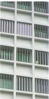
Distinctive sun-shading fins of Science Block
