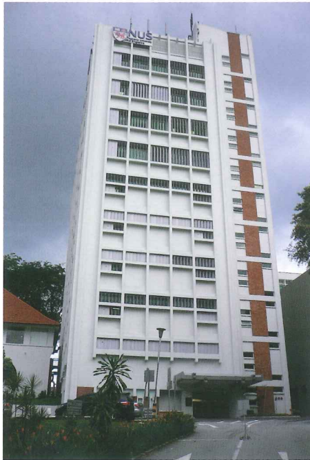
Science Tower refitted with trademark adjustable vertical sun-shading fins
