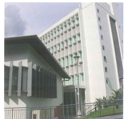
External shading fins of LT 1 retained
