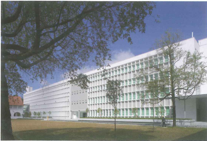
View of restored façade of Block B from quadrangle
