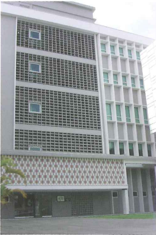
Entire original façade of Block B kept
