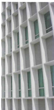
Deep concrete fins of Block B for effective sun-shading
