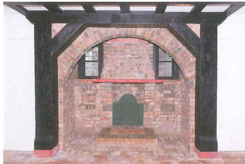
Fireplace and honeycomb-shaped terracotta floor tiles
