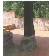
Timber column on stone base
