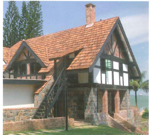
Secondary timber staircase to second storey
