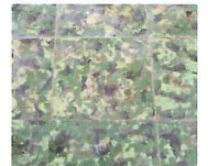
'Camouflage' floor tiles retained
