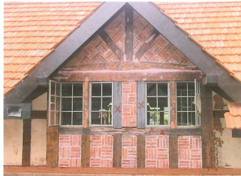
Timber elements and pilasters restored and painted black
