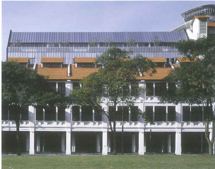
Restored shophouses with a distinctive new rear extension
