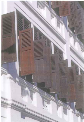
Original timber louvred windows reconditioned
