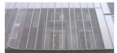
Condensing units well-integrated within rear façade
