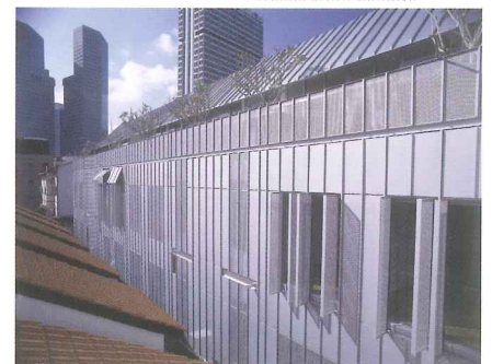
Modern treatment of rear façade contrasts against the conserved front portion
