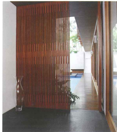
Entrance foyer with timber trellis screen
