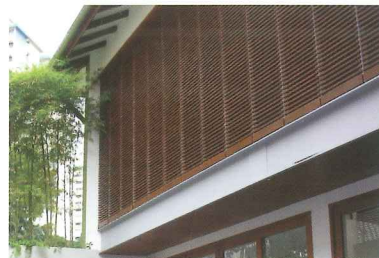
Timber louvered screen for shade, privacy and natural lighting
