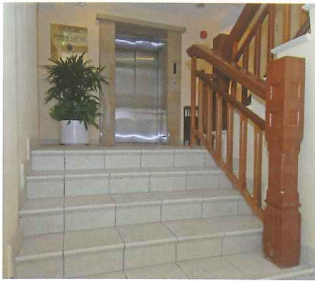
Modern lift sensitively inserted into staircase core
