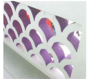
Art Deco fish scale detail at balcony parapet
