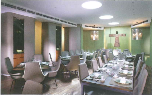
Pool's porthole glass base as skylights to restaurant
