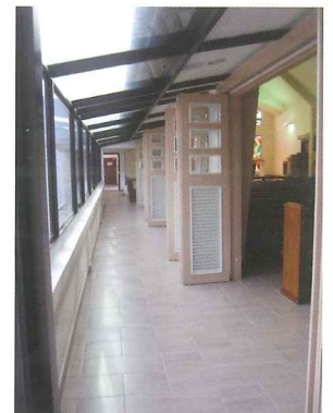
Clear glass skylight sensitively added to verandah flanking main sanctuary
