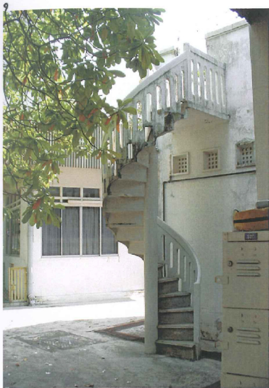
9 Spiral staircase at the rear of the church
