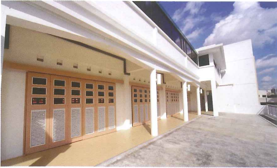
Folding accordion doors kept
