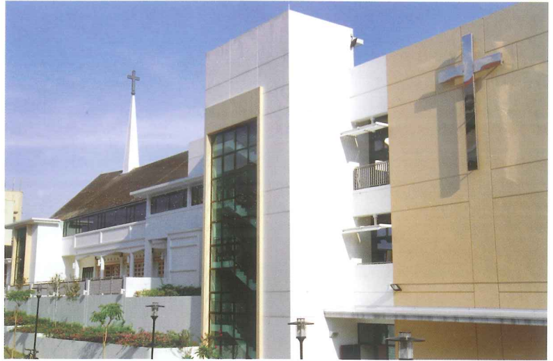
New annex block sensitively added to west side of building
