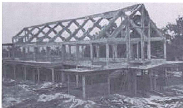
The church building under construction
