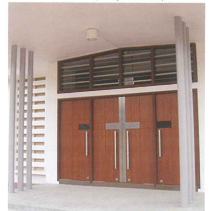
New front doors in matching stained timber
