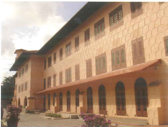
Restored façade repainted to match original colours
