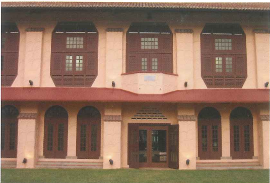
Distinctive polygonal timber framed windows and balcony kept
