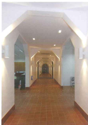
"Petal-shaped" beams intentionally exposed
