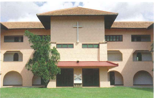
Three-storey Restroom Block converted into a meeting/gathering space
