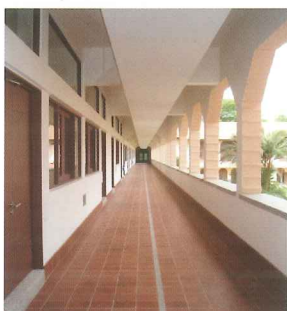
Queue lines and floor tiles along corridor kept
