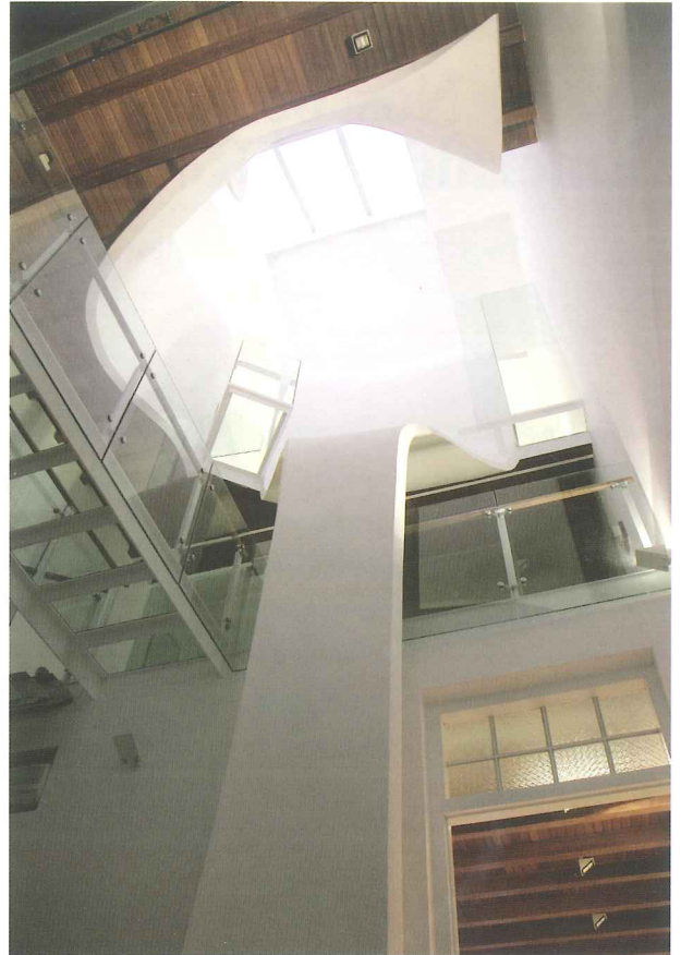
Sculptural light reflector and glass link bridges at Unit 63
