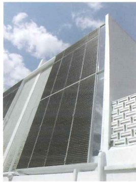
Rear façade with screening
