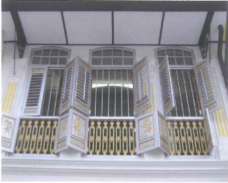
Ornate details of the front façade sensitively restored
