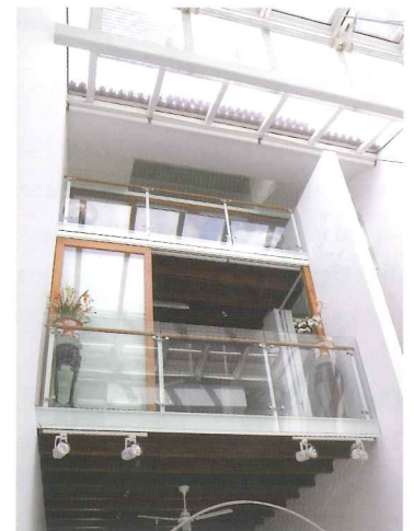
High volume air-well with retractable glazed panels at Unit 65
