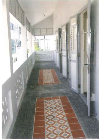
Original patterned floor tiles reused as decorative inlays at balcony
