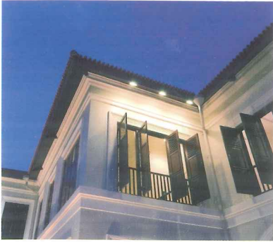
Night lighting enhances the details of the restored building
