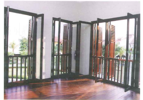
Secondary windows added to existing French windows at the upper storey for air-conditioning purposes
