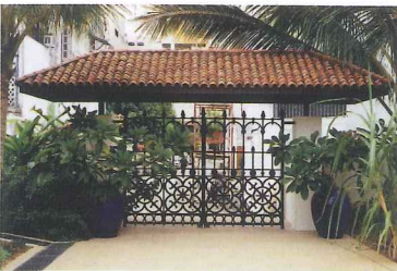
Original roof tiles reused at side entrance gate
