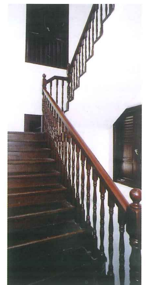
Restored hardwood staircase with handrails
