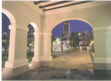
Arched entrance porch restored
