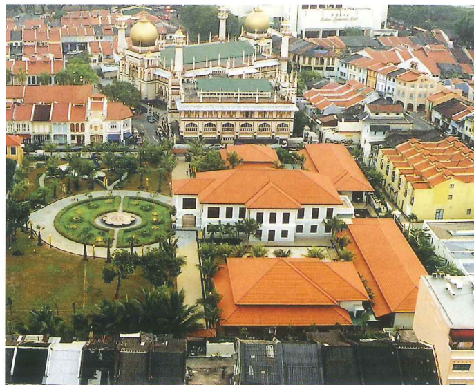
Aerial view of the museum complex in the heart of the Kampong Glam Historic District
