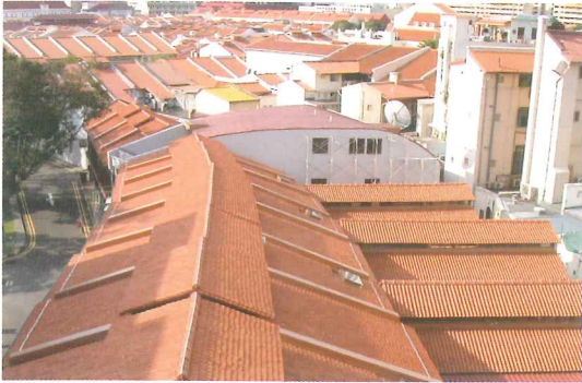
Barrel vault roof of new infill development at Unit 15 adds interest to the traditional roofscape of the area
