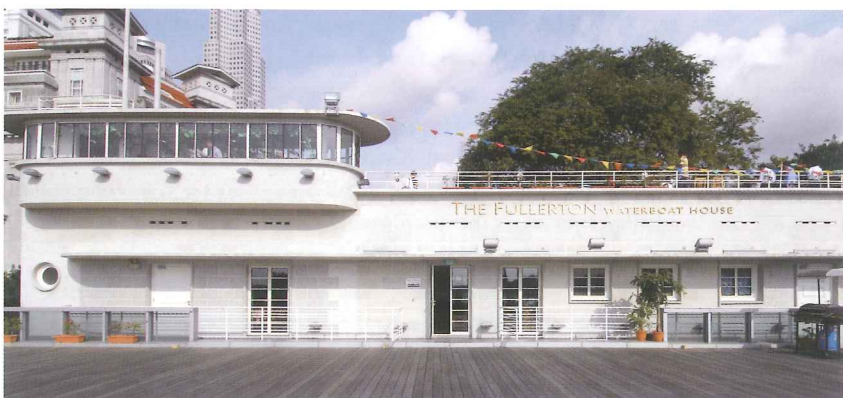
Timber decking at the roof of the new extension enhances the conserved nautical rear façade
