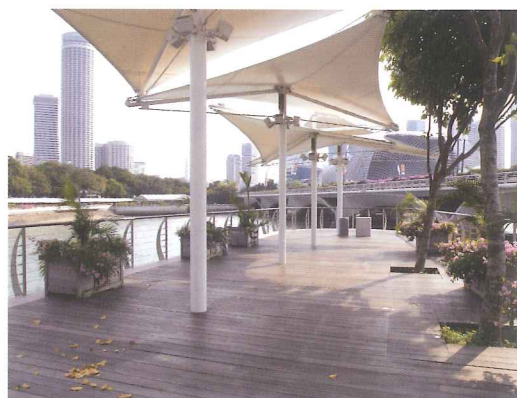
New timber pier deck at old Merlion site
