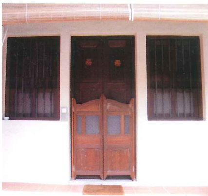
First storey front façade
