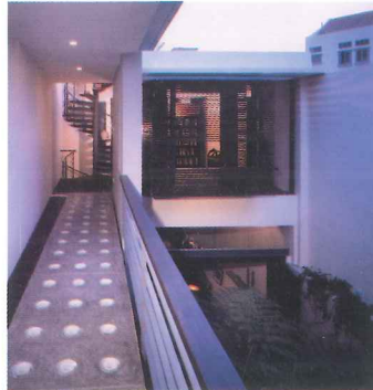
Light weight glass block bridge between the old and the new
