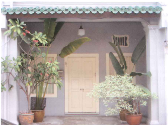
Front façade retained and restored
