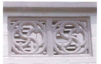
Pre-cast concrete vents
