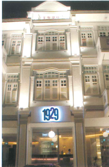
Restored to a hip boutique hotel
