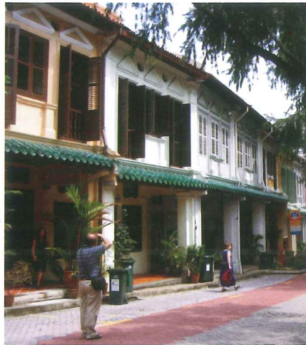
Peranakan terrace house restored for gracious living
