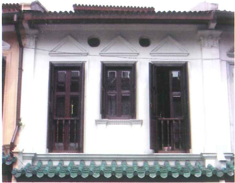
Second storey front façade with geometric detailings
