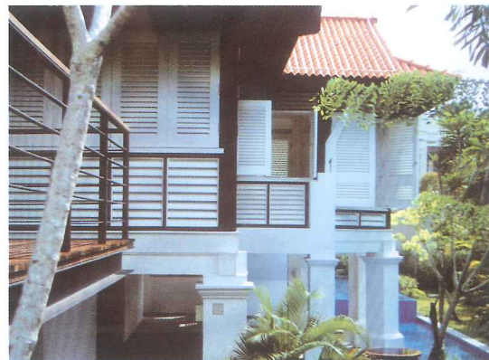
Restored first storey verandah
