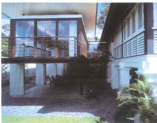
New single-storey extension
