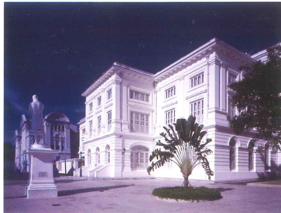
Architectural treasure adapted for reuse
