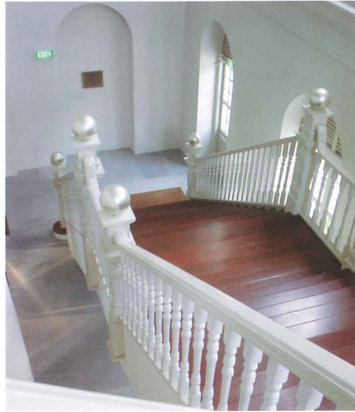
Original timber balustrade at central staircase
