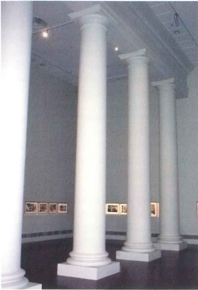
Circular masonry Doric columns
