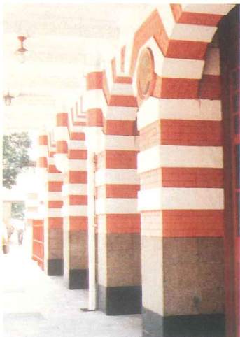
Rusticated red brick and plaster banded façade restored
