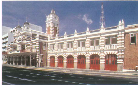
Old fire station rejuvenated
