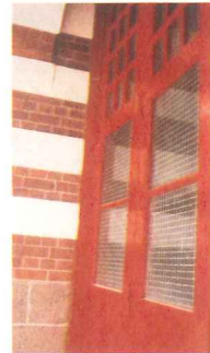
Original arched timber door restored
