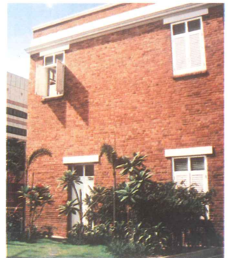
Side external façade restored to original
