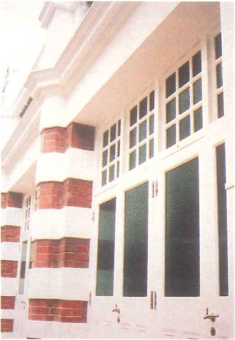
Timber framed doors with glass infill
