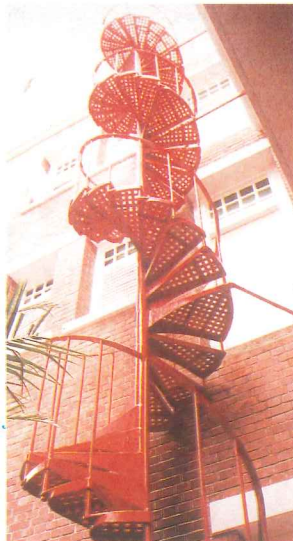
Spiral staircase with wrought iron handrail and balustrade
