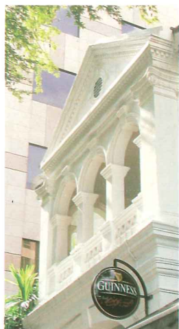
Second storey verandah with pediment and decorative balustrades
