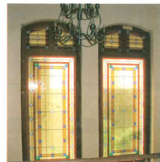
Stained glass secondary windows added
