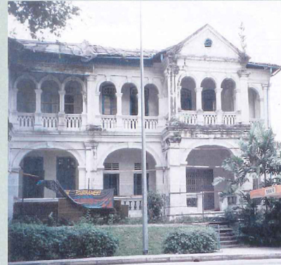
front facade of existing building
