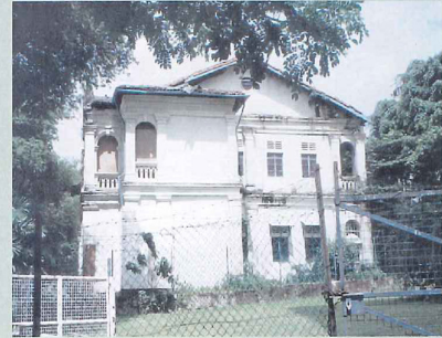
side facade of existing building
