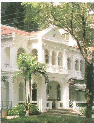
Main entrance with new flight of steps and planter boxes
