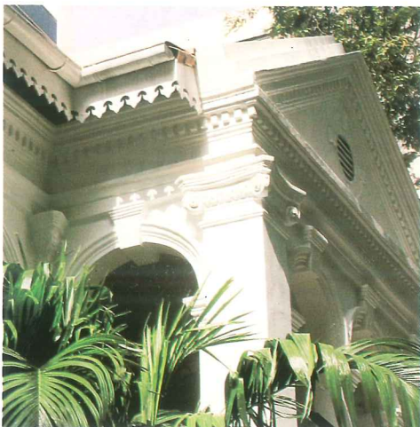
Corner details showing decorative timber fretwork and column capitals
