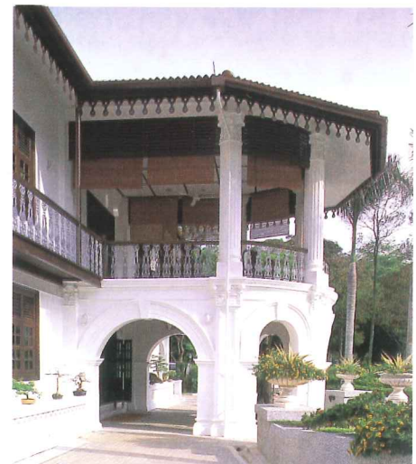
Entrance porch and front balcony retained
