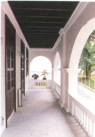
South verandah at 1 st storey
