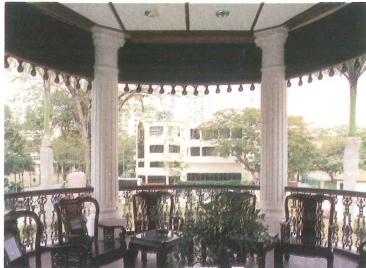
Original ambience of open sitting area at balcony retained
