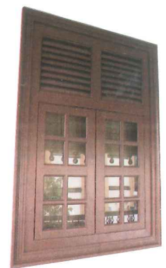
Timber framed windows restored
