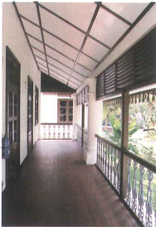
Open side verandah with timber flooring
