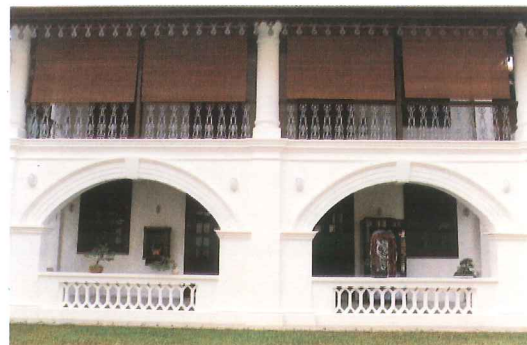
Classical arches with moulded architrave and decorative parapet walls restored
