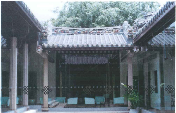
FIRST COURTYARD AFTER RESTORATION
