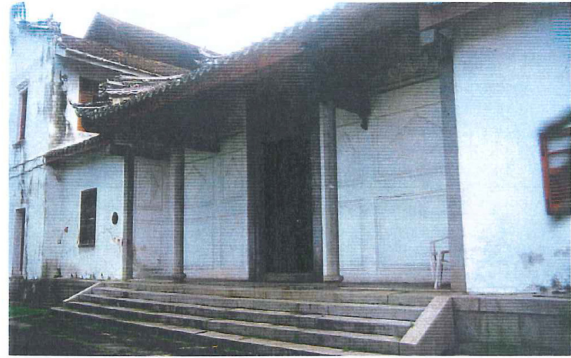
VIEW BEFORE RESTORATION
