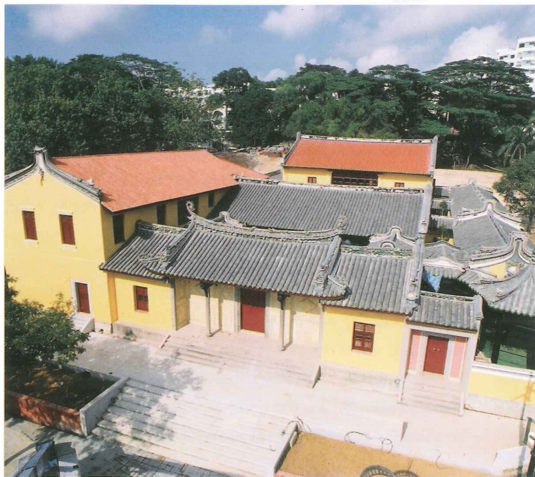
Aerial view of the restored building
