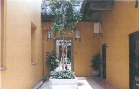
NORTH WING CORRIDOR AFTER RESTORATION
