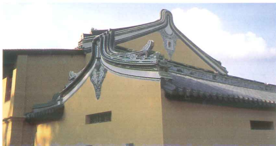
Gable end walls with fine artworks
