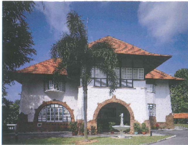
A sensitively restored bungalow
